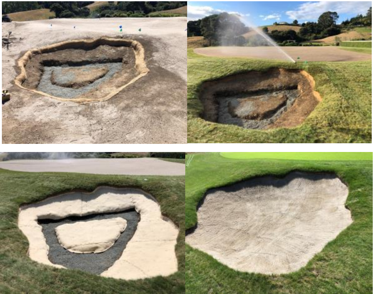
Figure 8. Drainage and liner installation process in a bunker.
