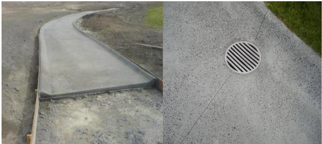
Figure 12. Cart / maintenance path installation.
